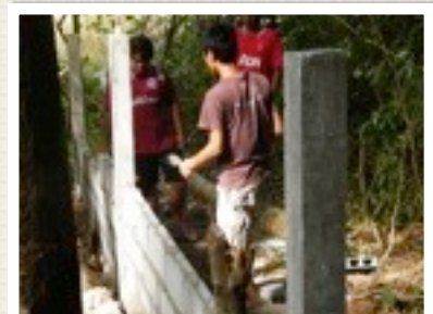
BANGKOK TEAM WORKING ON OUR HOUSE IN THE VILLAGE
